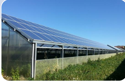
PV system on greenhouse
